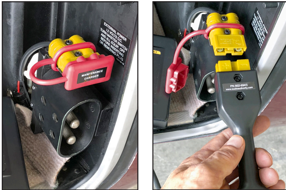
Figure 5. Finished installation example.
